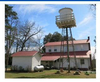
.The **Water Tower** used to provide water to the Main House and the farm. Water was drawn from the nearby well and originally flowed due to gravity, but an electric pump was installed in the 1940's. The farm's water supply was then stored in a pressurized tank next to the **Well House**. Inside the Well House, visitors can peer down into Andalusia's 30–foot deep, brick–lined, hand–dug well.
