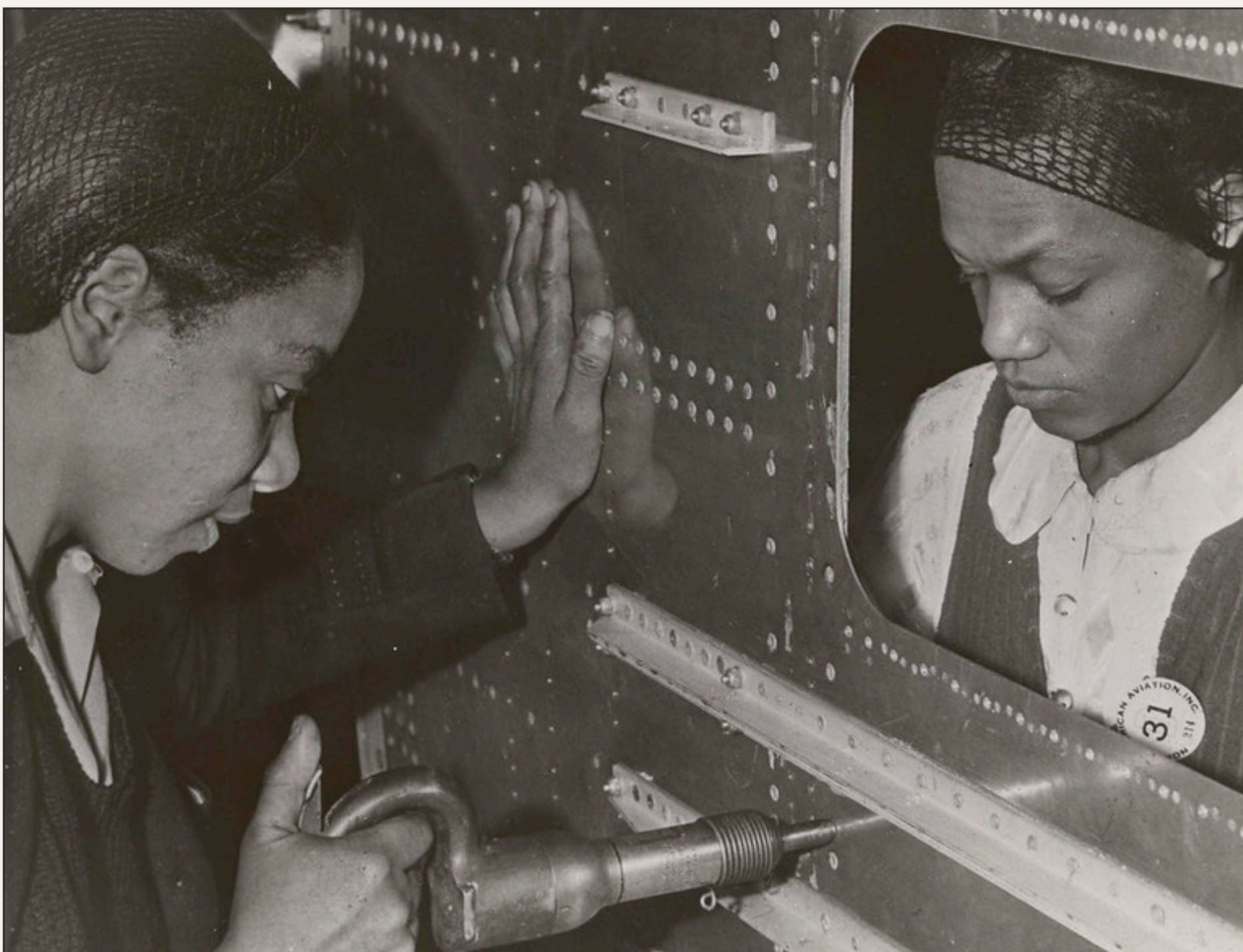
“Evelyn T. Gray, Riveter and Pearlyne Smiley, Bucker, Complete a Job on Center Section of a Bomber.” Courtesy of the National Archives.
