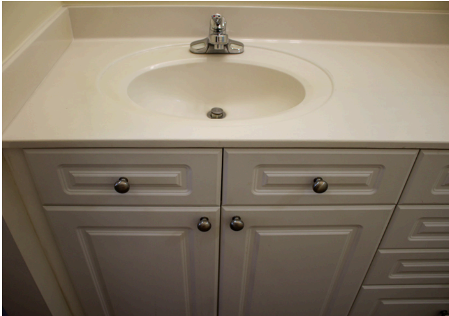
Bathroom Sink and Cabinets
